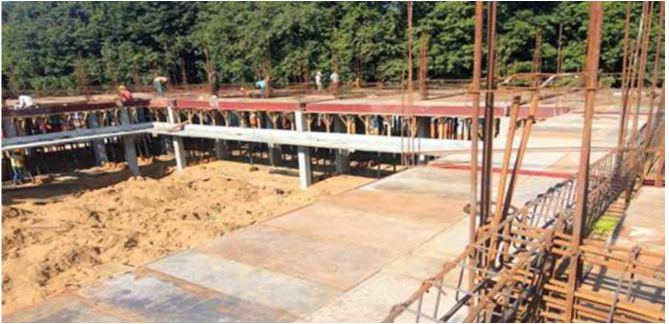
Ongoing Construction works
